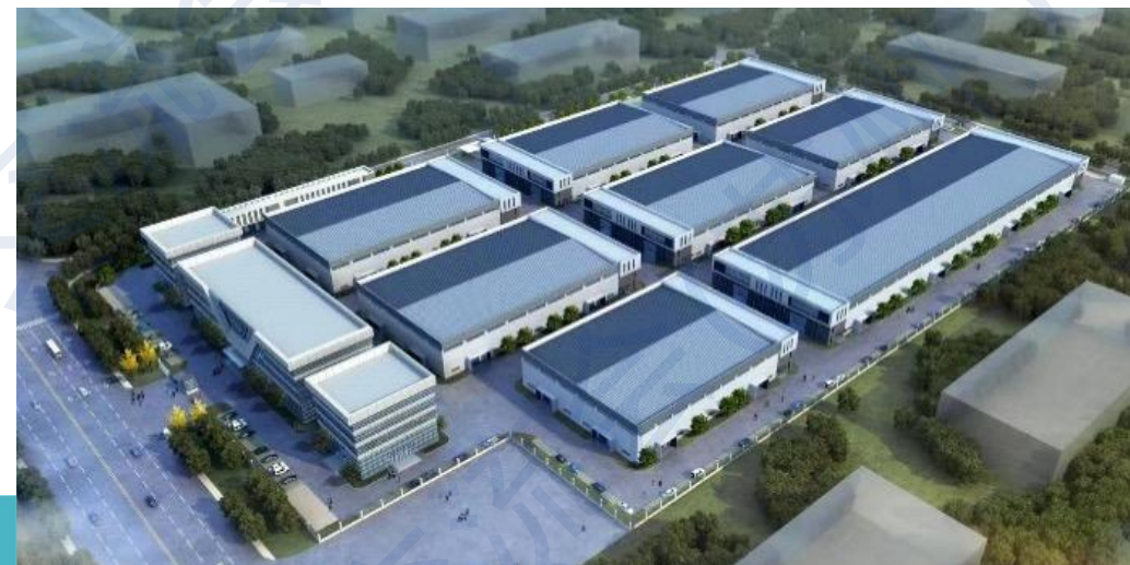
80,000m 2 for R&D labs and scale-up facilities
